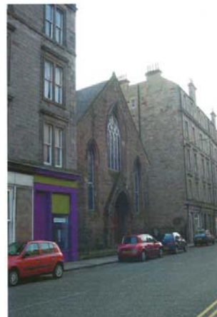
Duke St before demolition
