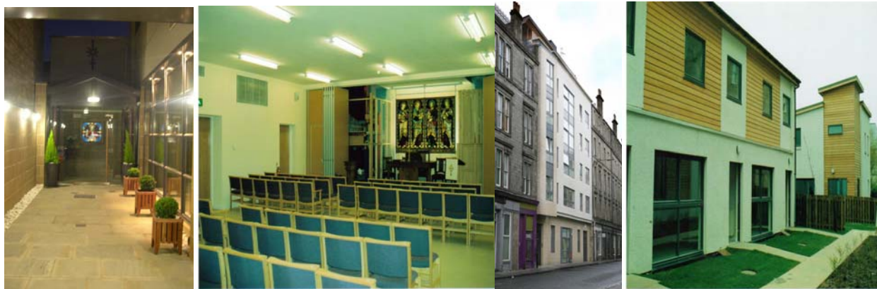
The new church centre entrance and sanctuary; the street front with flats above and the family homes at the rear
