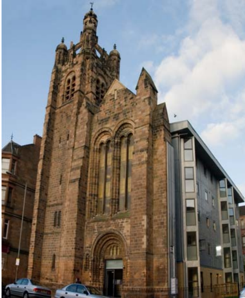
Strathbungo former Church of Scotland, Glasgow
